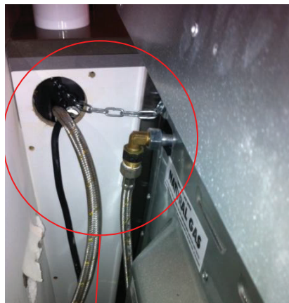
Hole in cabinet is too large, allowing the upright cooker to tilt forward
